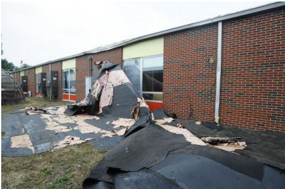
July, 2012: A 2,200 square foot section of the Christopher Elementary School roof was ripped off of the building during storms Sunday. As a result a number of classrooms were damaged by flooding.
