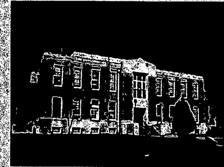
Hamilton County Courthouse
